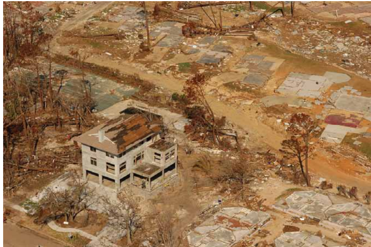
Hurricane Katrina August 2005 - $108 billion in damages, 1,833 lives taken. ICF home survives the storm.
